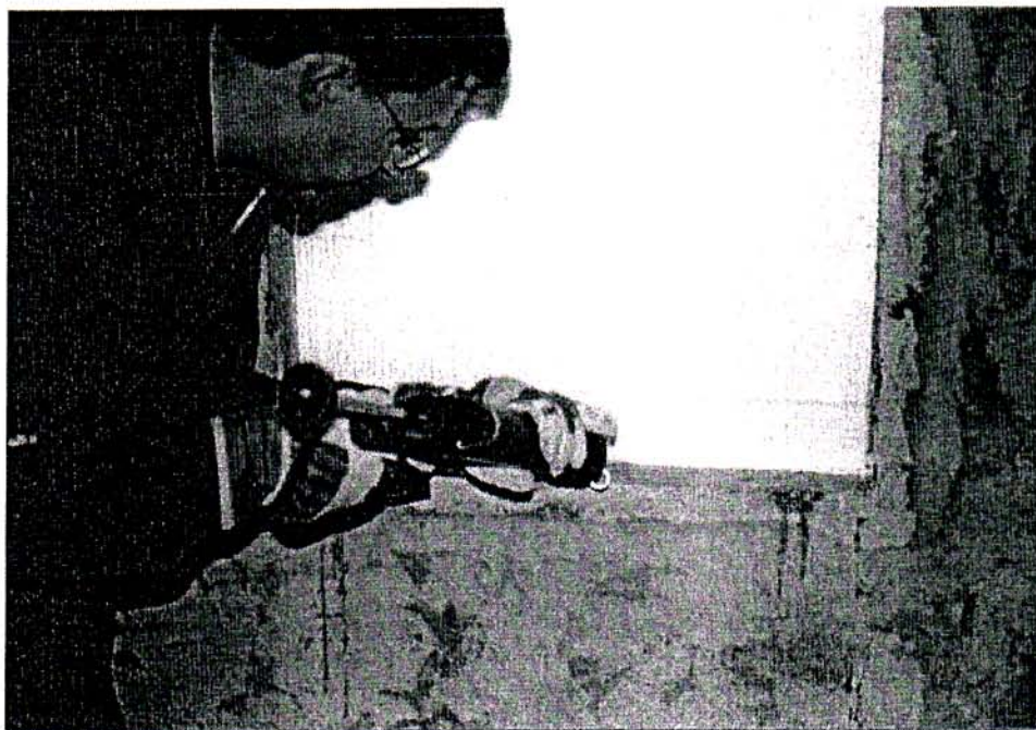
Figure 5: Frame joint being sealed with sealant Hilti CP 606
